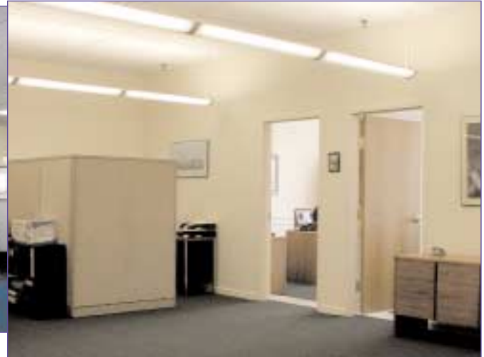
Pega's new space uses effective, energy-efficient lighting.
