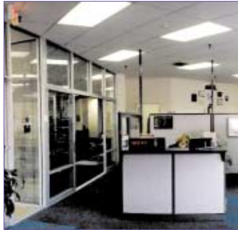
Non-energy-efficient lighting was used in Pega's old office space.
